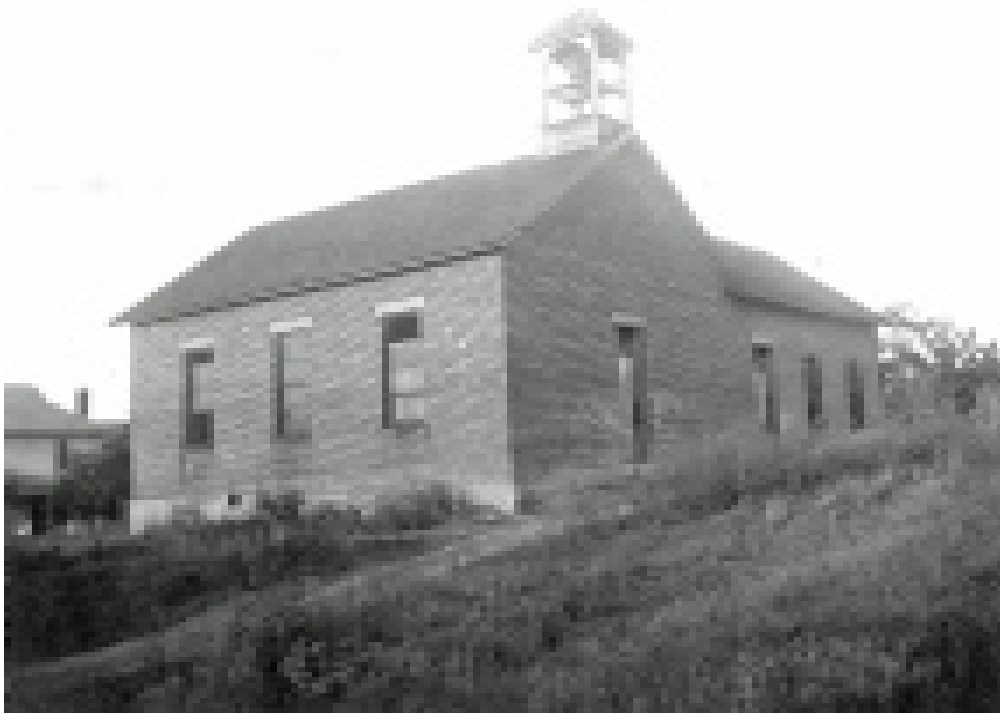
Jerome brick school house, built in 1860; located just north of Ryan Memorial school site on Jerome Road.
